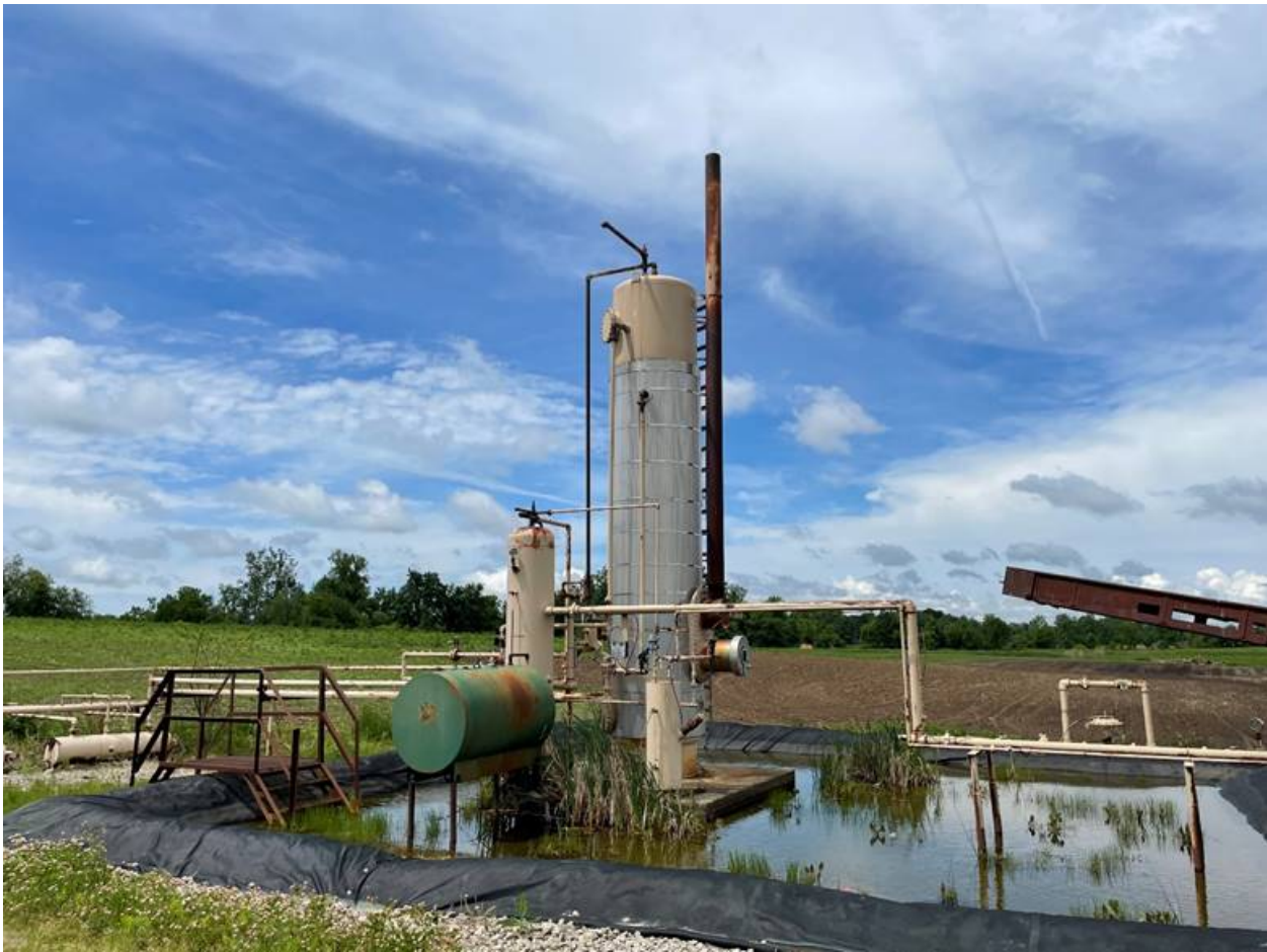
Image 14: Lindeman 1-36 heater treater and line heater.
