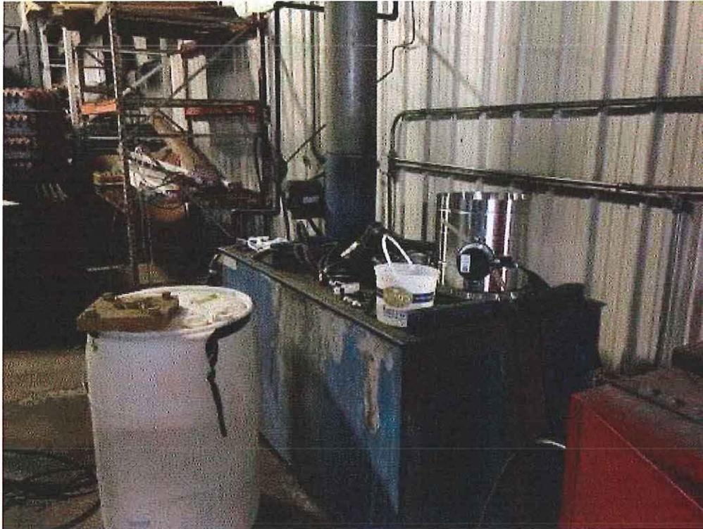
**Image 9(Evaporator)** : Natural gas-fired wastewater evaporator for wash bay.
