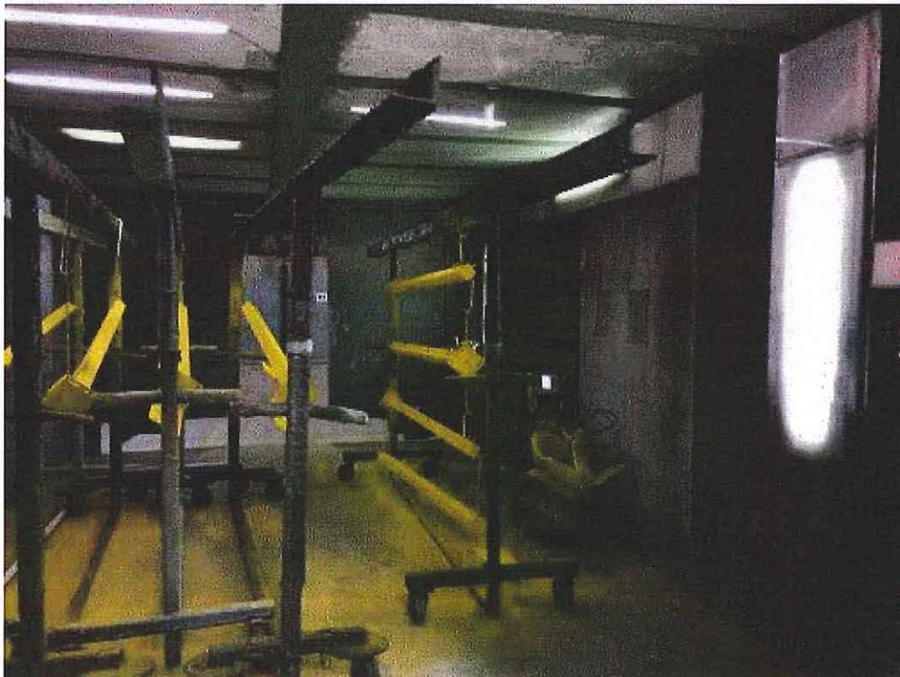
**Image 6(Powder Coating)** : Powder coating booth with cartridge filters.
