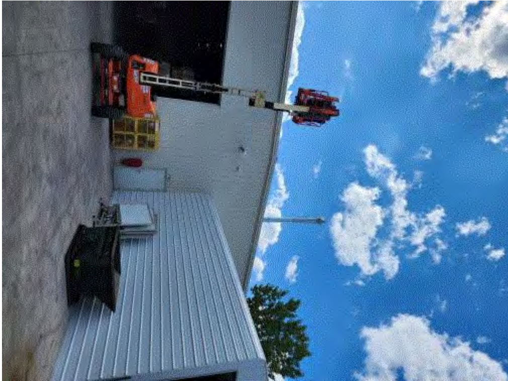
Image 3(Post-Install) : Photo Credit: Cleanlites. Stack height is post-install of the 5' extender.
