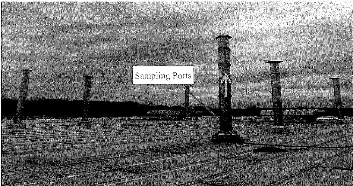
**Figure 2-5 Post Quench Washer Sampling Location**
