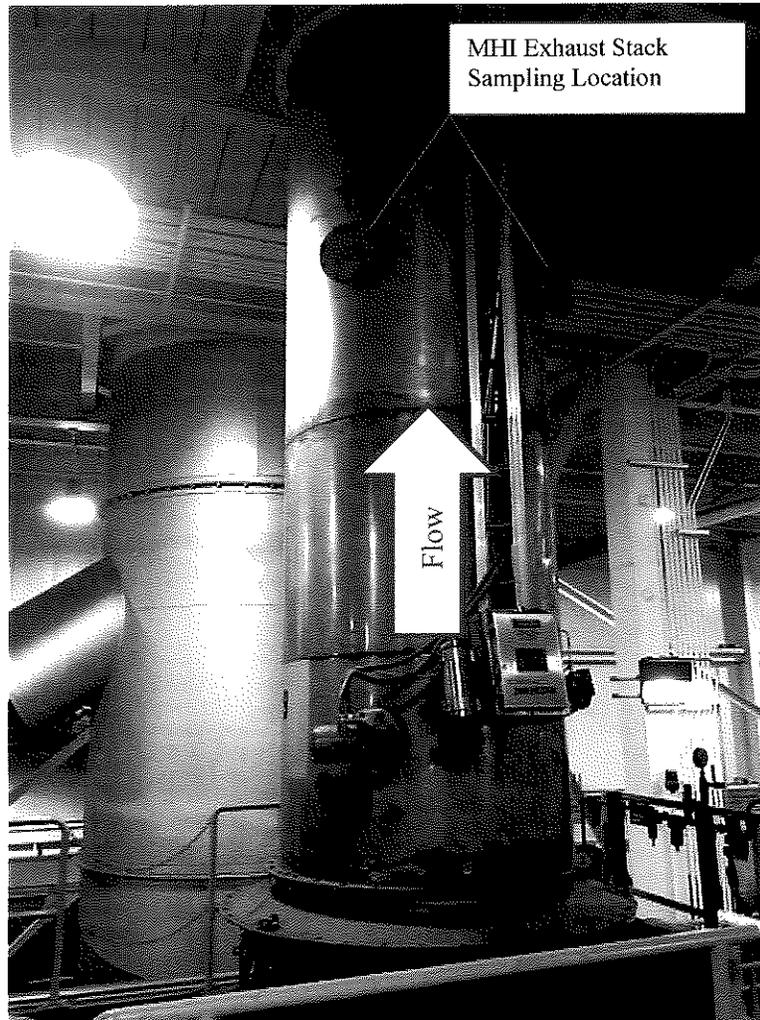
**Figure 2-1. Incinerator Sampling Location**
