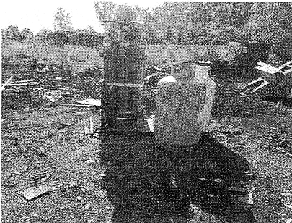
**Image 6(Torch cutting)** : Torch cutting area with portable oxygen/propane tanks.
