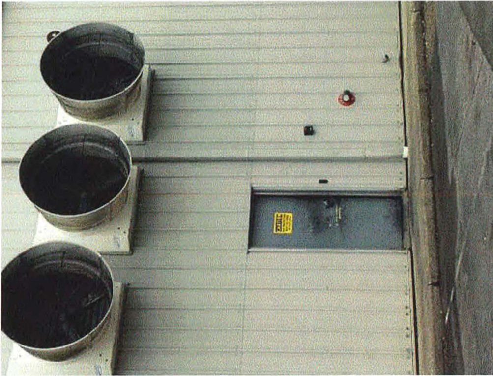
Image 1(Wall Exhaust Fans) : Exhaust fans above entrance - note black particulate collected in each well
