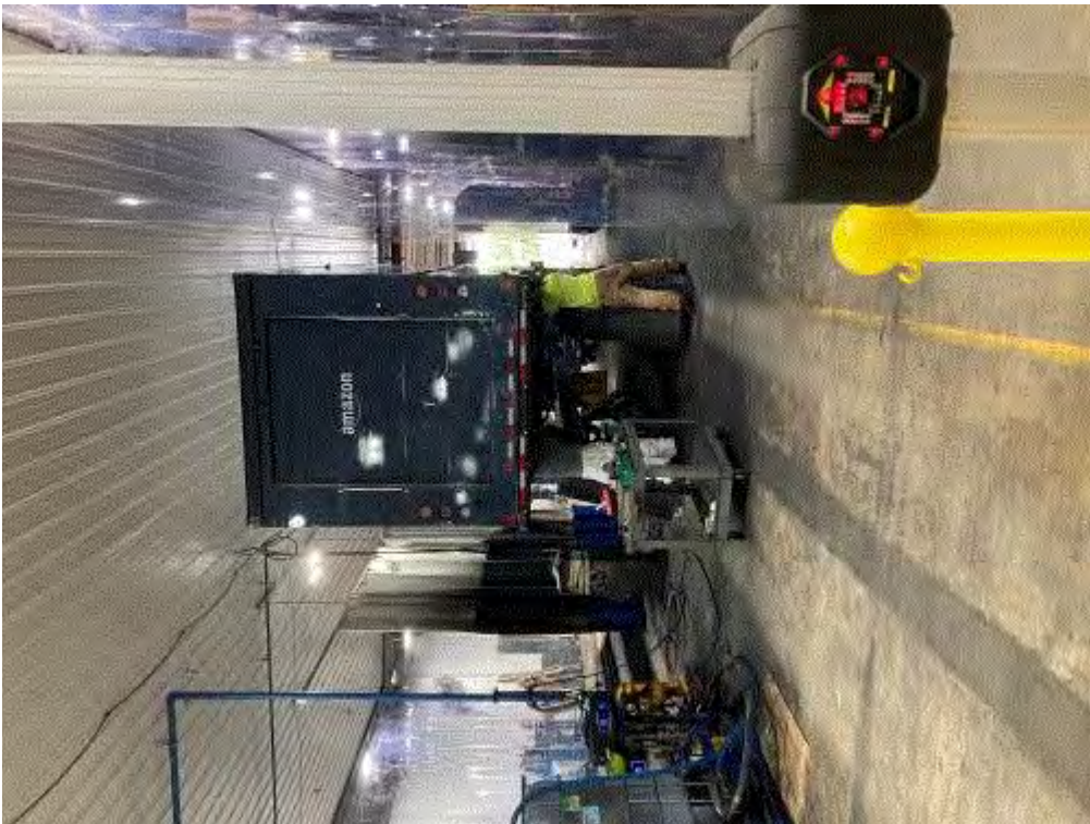
Image 3(Undercoat) : Undercoat "booth" area. Note plastic sheeting on either side and bay door open. Plastic sheeting to be installed on front and rear also.
