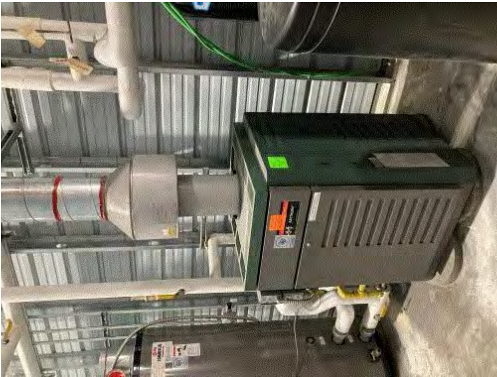
Image 2(Boiler) : Boiler used to heat the wash water in the paint prep wash booth
