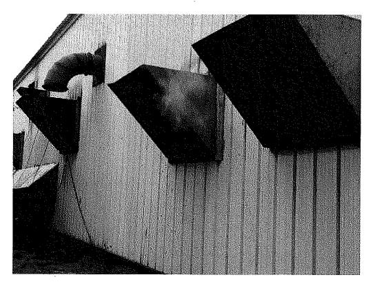
Image 4(BPV Environmental) : Baghouse exhaust points - Dust is from the cleaning of BH 407.
