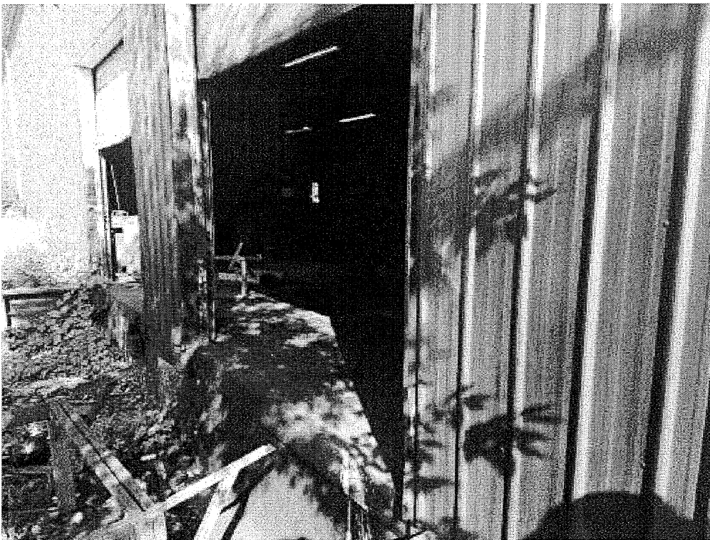
Image 6(Bay doors) : Bay doors to coating area with overspray on walls.
