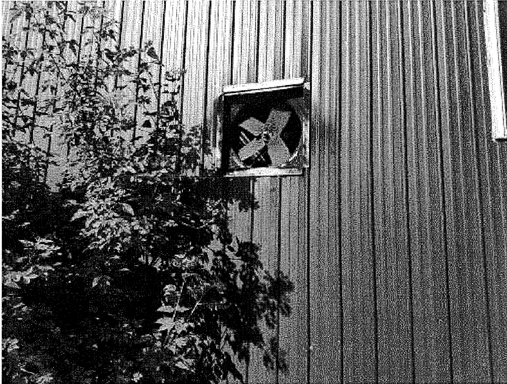
Image 5(Exhaust fan) : Side wall exhaust fan exterior view
