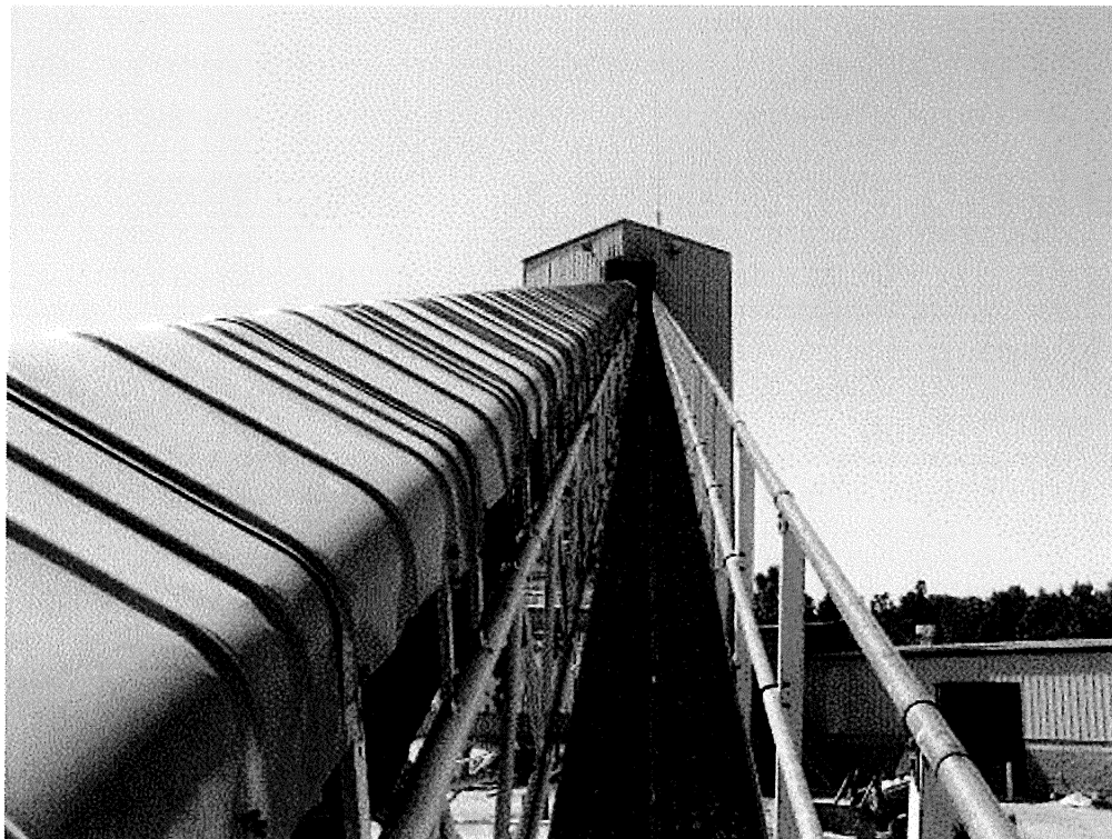
Image 2(002) : Catwalk to top of batch plant.
