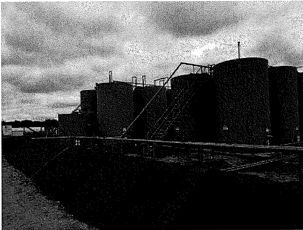
Image 3(Oil/brine storage) : Oil/bring storage tanks.
