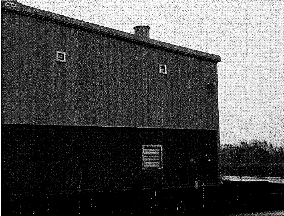
Image 6(New Incinerator bldg) : New incinerator building showing incinerator exhaust stack.
