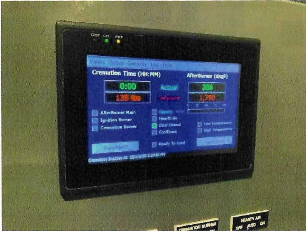
**Image 1(Main Control Panel)** : Main control panel displaying the secondary combustion chamber temperature, setpoint temperature, and stack opacity.
