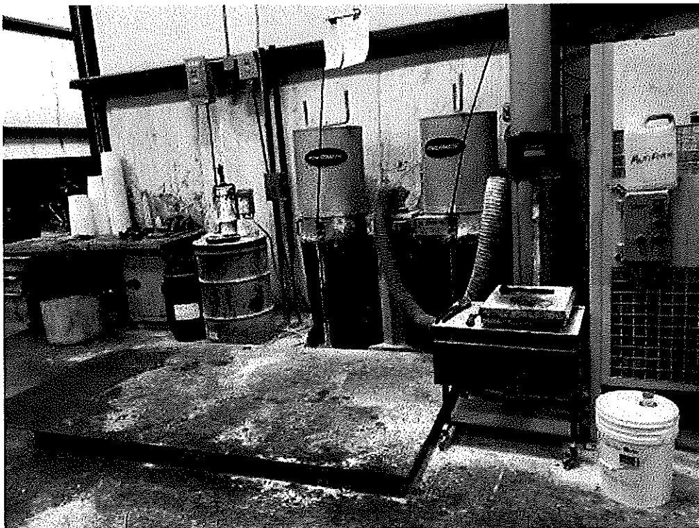
Image 6(8) : Powder mixing station with dust collection
