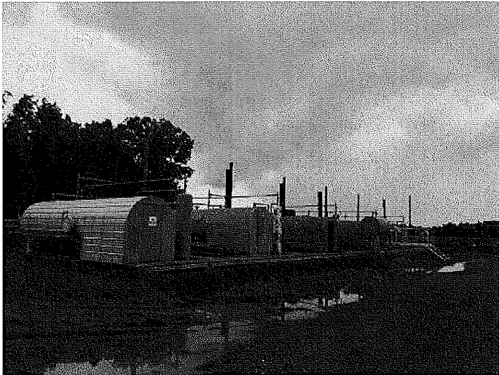
Image 3(Heater treaters) : Heater treaters
