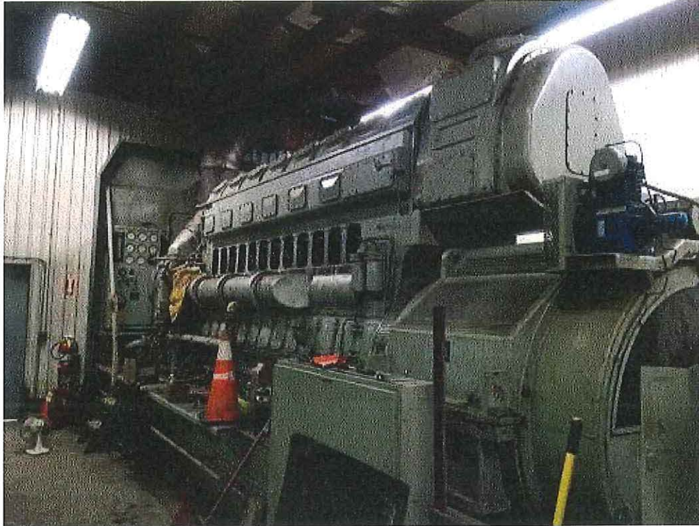
Image 1(Unit #1) : Fairbanks-Morse 12-cylinder opposing piston diesel engine.
