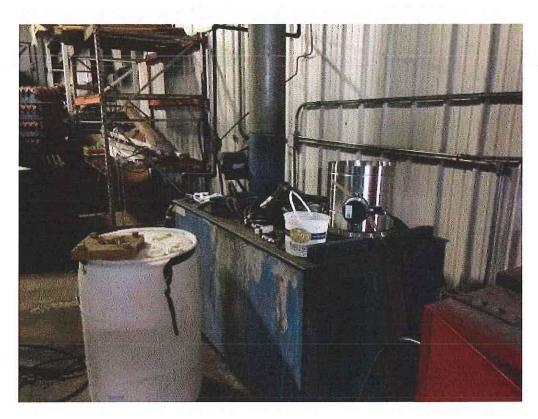
Image 9(Evaporator) : Natural gas-fired wastewater evaporator for wash bay.
