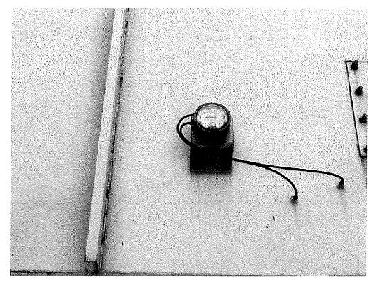
Image 3(Magnehelic) : Magnehelic pressure drop gauge reading 7" WC.
