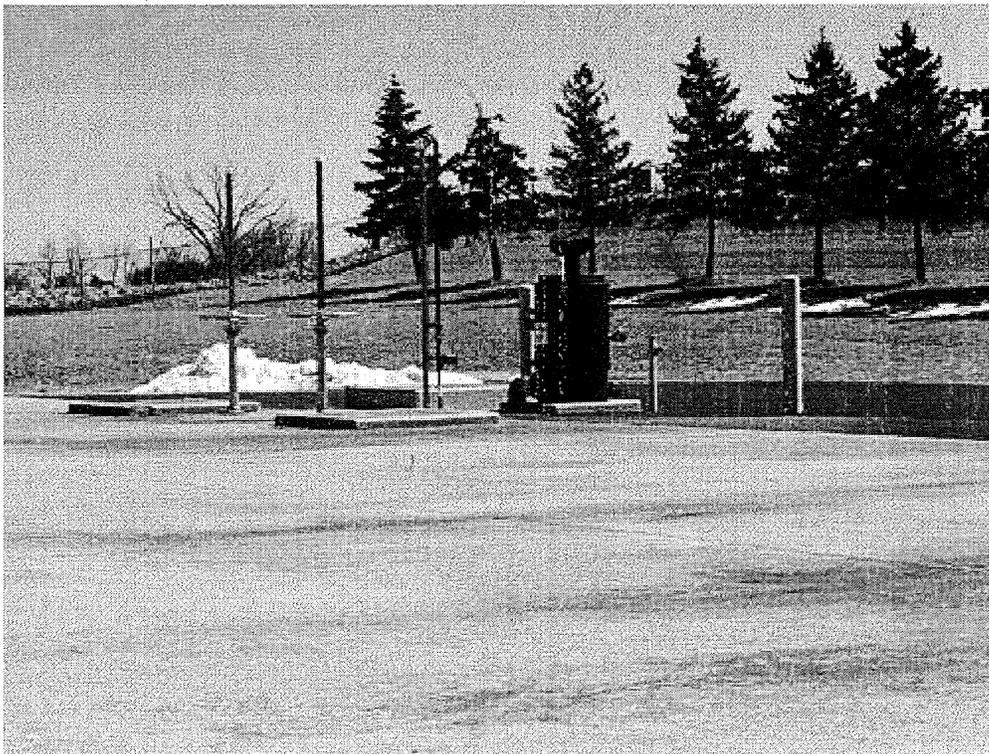
**Image 1(Gravity fed carbon)** : This is one of two passive, gravity fed carbon canister that controls for odors on
