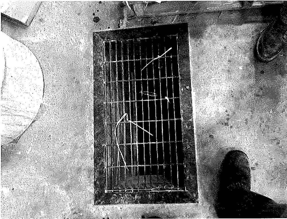
Image 5(Floor vent) : One of the floor vents that exhaust to a 40 foot stack
