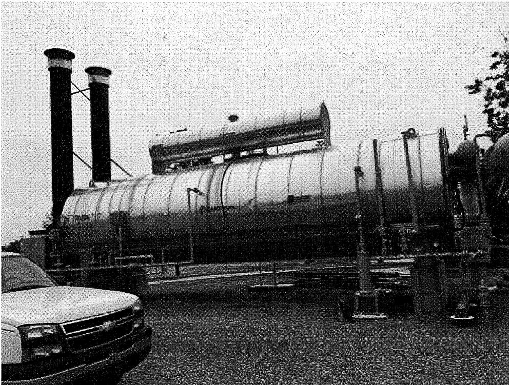
**Image 7(Line heater)** : A 13 MMBtu/hr line heater.
