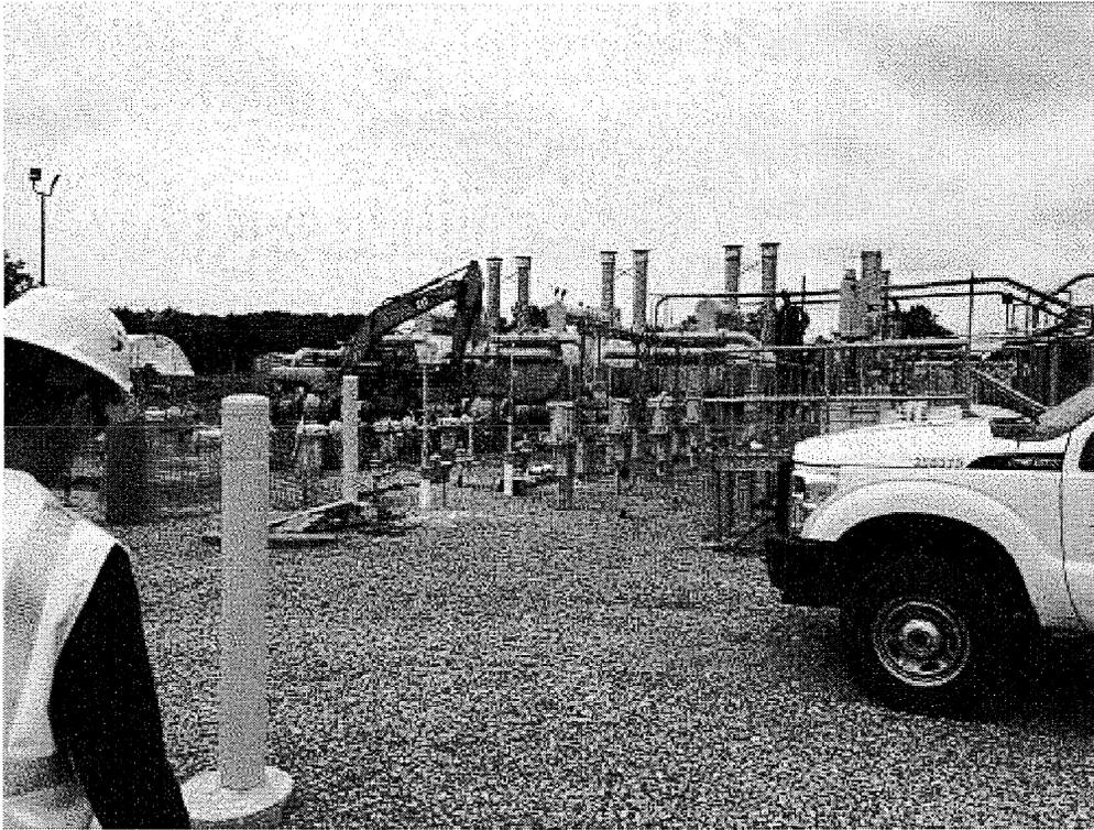
**Image 8(Line heaters)** : Three 14 MMBtu/hr line heaters.
