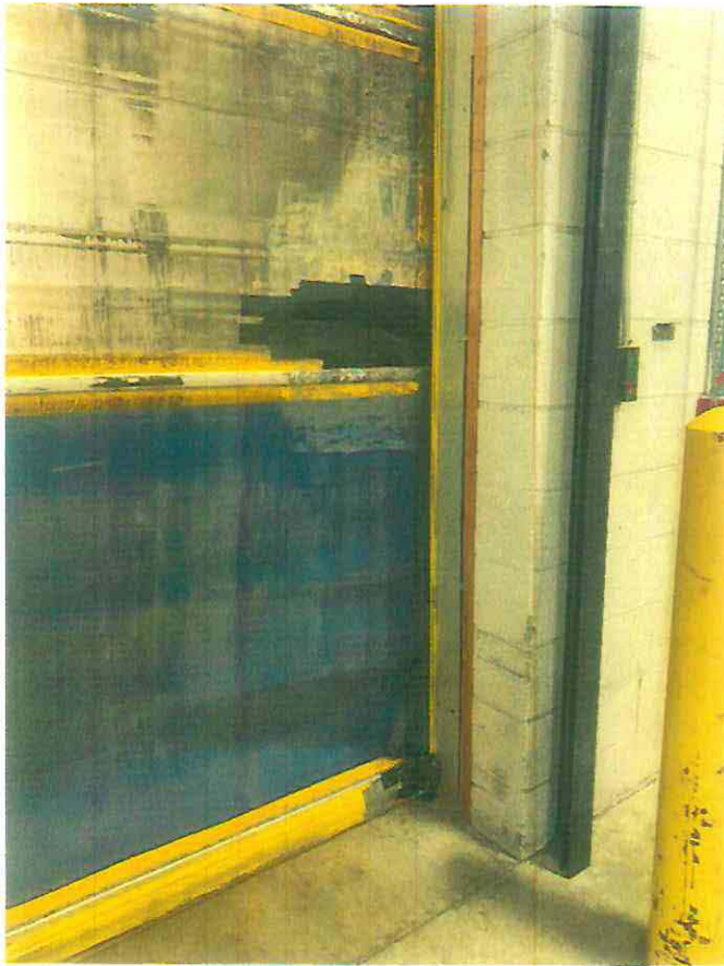
Above: Photograph of repairs to door on December 20, 2022.
