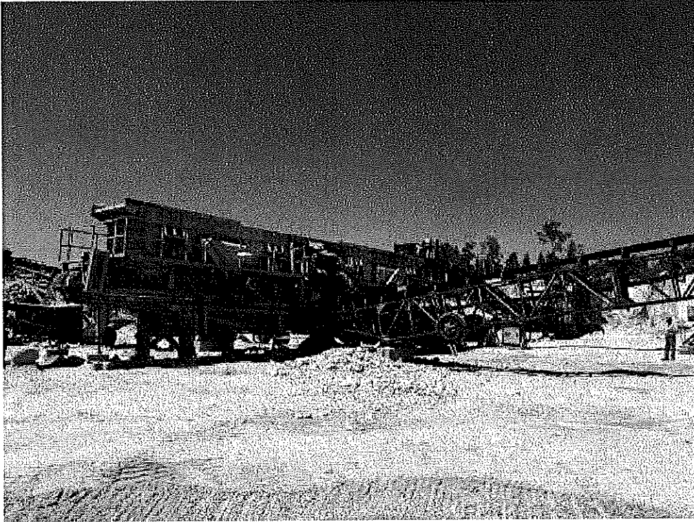
Image 5(Crusher Plant) : Can Agg, Inc. portable crushing plant at Simmons Pit.
