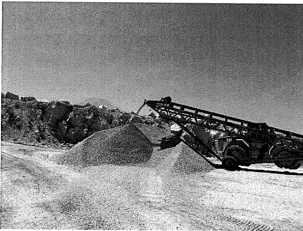
Image 4(Transfer Point) : Transfer point from conveyor to stockpile.
