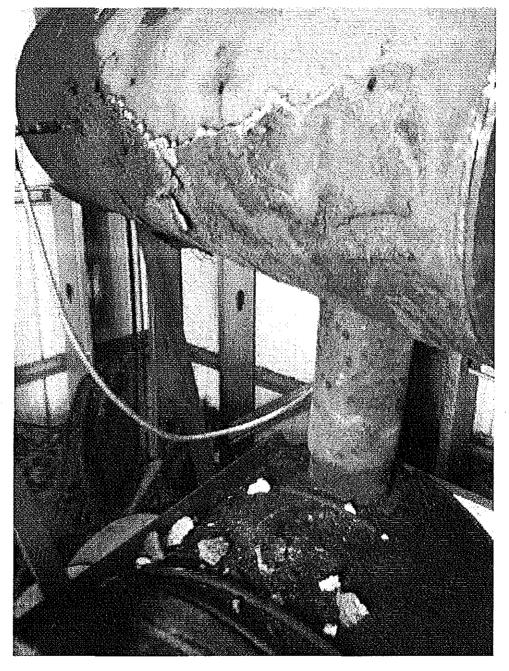
Image 4(ccvc4) : jacket disintegration on afterburner
