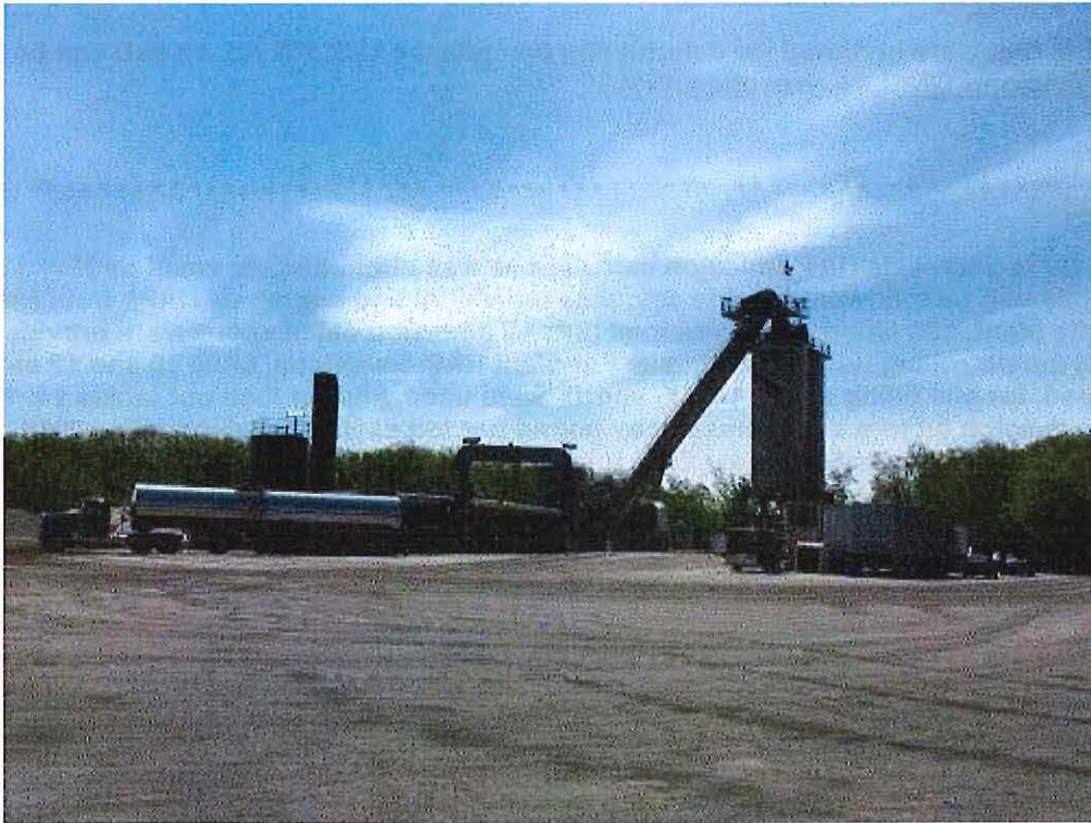
Image 1(HMA Plant) : Payne & Dolan Plant C34
