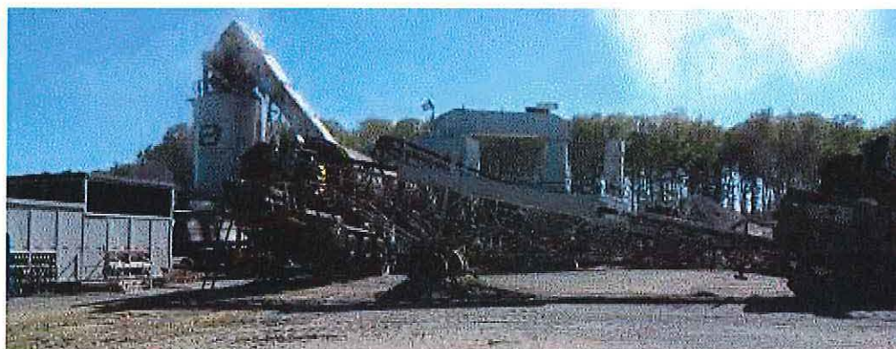
Image 2(C342) : Silo, drum, conveyors
