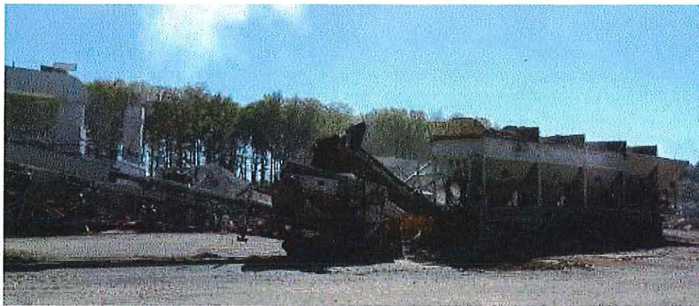
Image 1(C341) : Bins and conveyor
