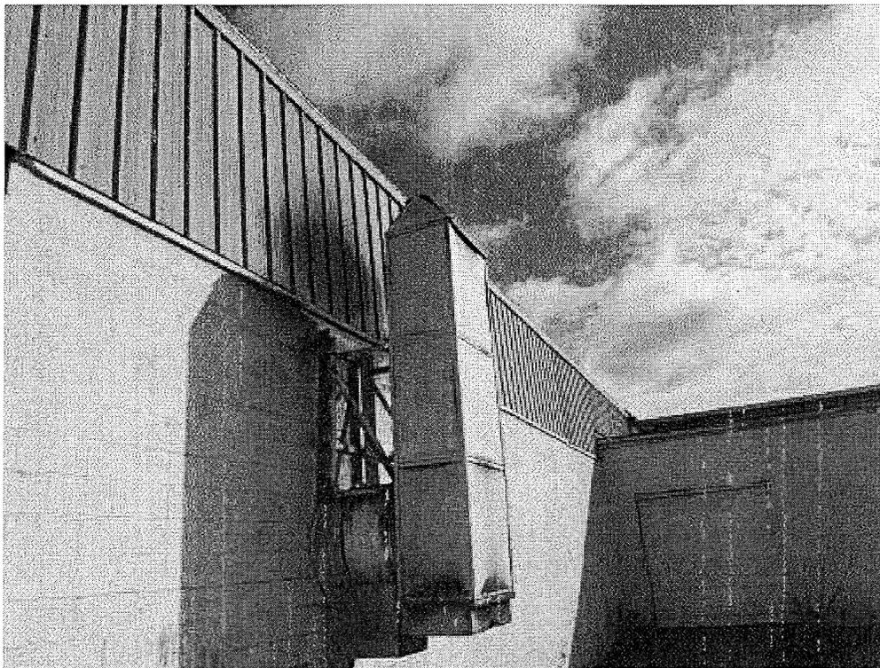
**Image 6(paint booth exhaust)** : Paint booth exhaust stack. Note overspray on the building wall.
