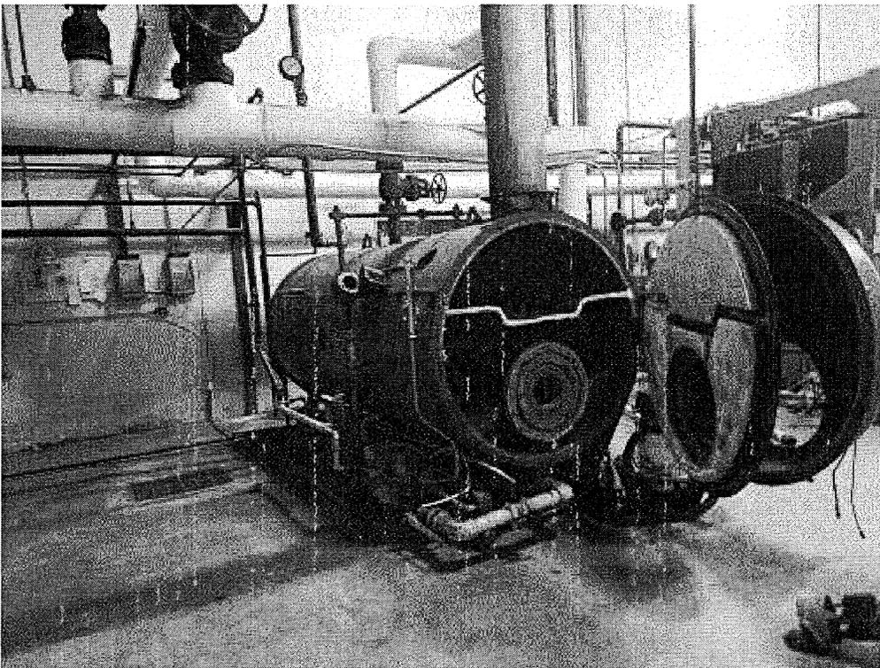
**Image 2(Boiler)** : 100 HP natural gas fired boiler built in 1972.
