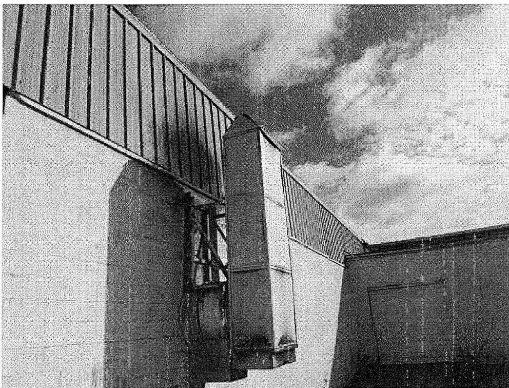
**Image 6(paint booth exhaust)** : Paint booth exhaust stack. Note overspray on the building wall.
