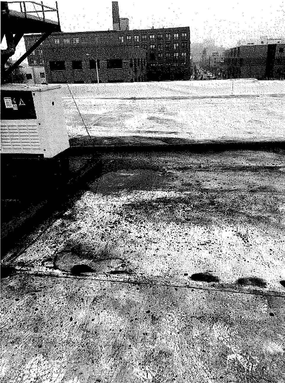
Image 2(EUBASECOAT #2.2) : Improper control of paint particulate.
