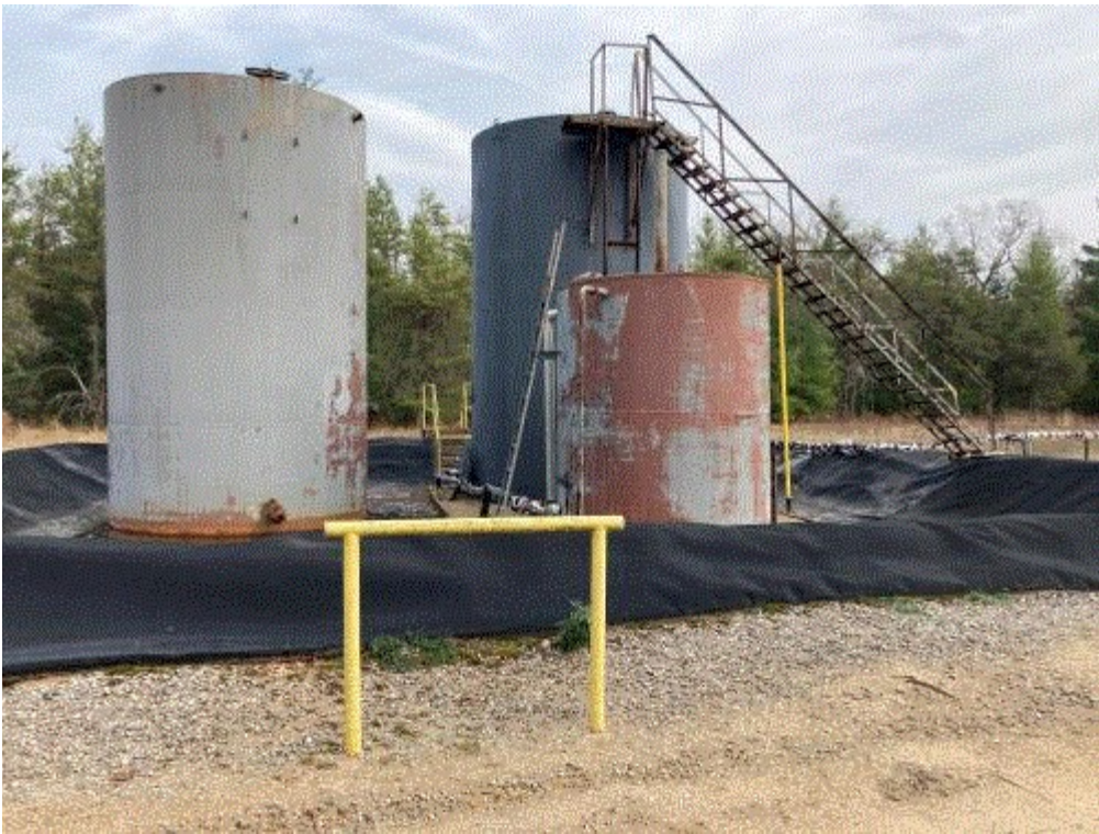
Image 2(3 AST Tanks) : 2 Brine Tanks and 1 Slop Tank - all meet exemptions.
