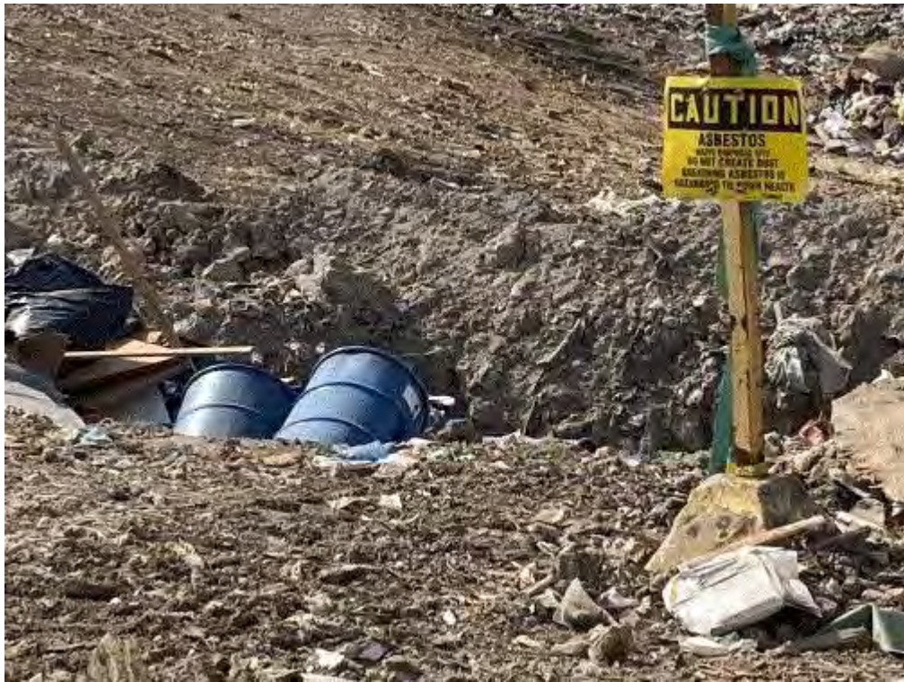
Image 3(Asbestos Close-up) : Close-up view of items disposed in asbestos trench
