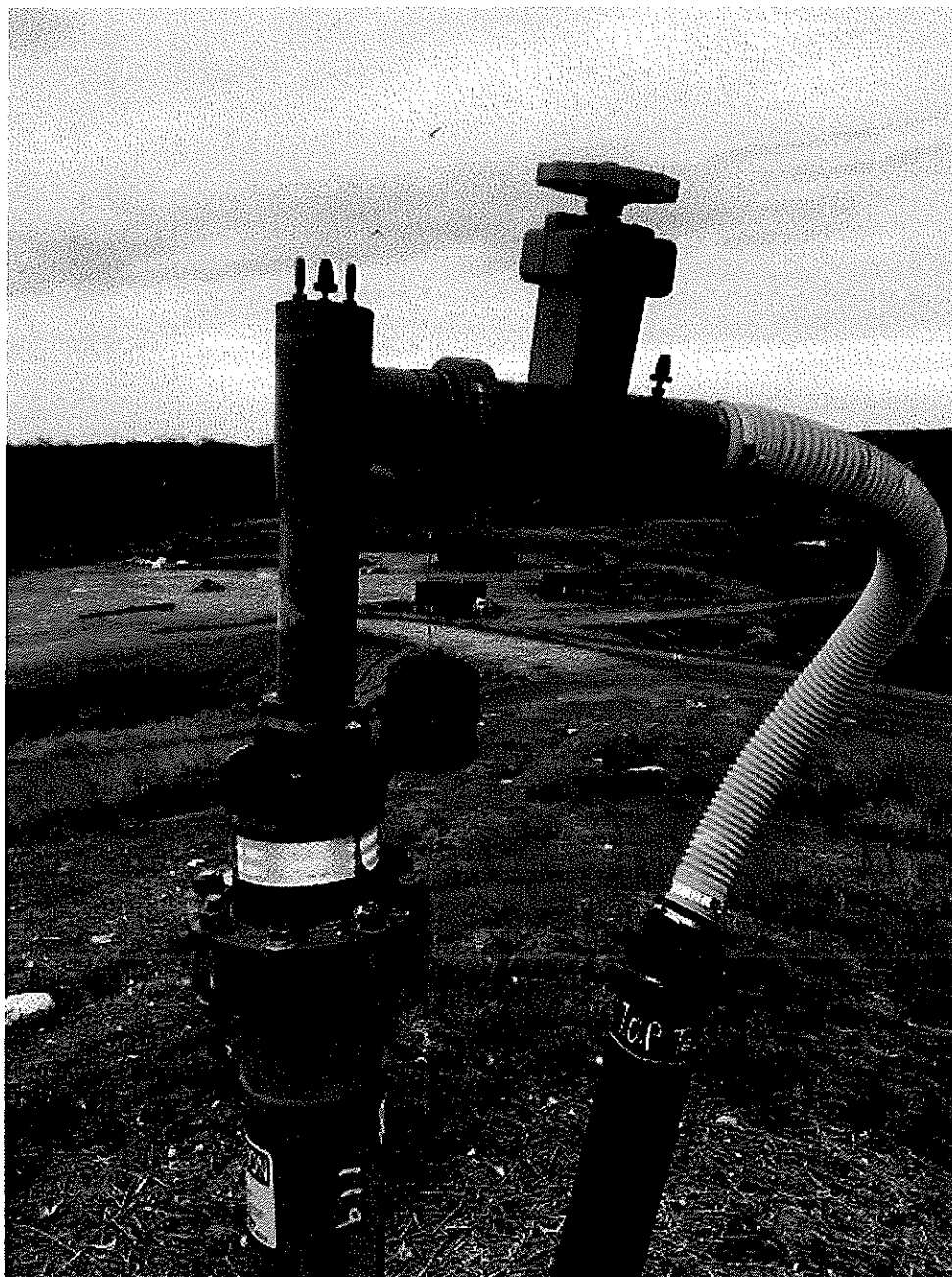
Image 5(9) : Landfill gas well riser
