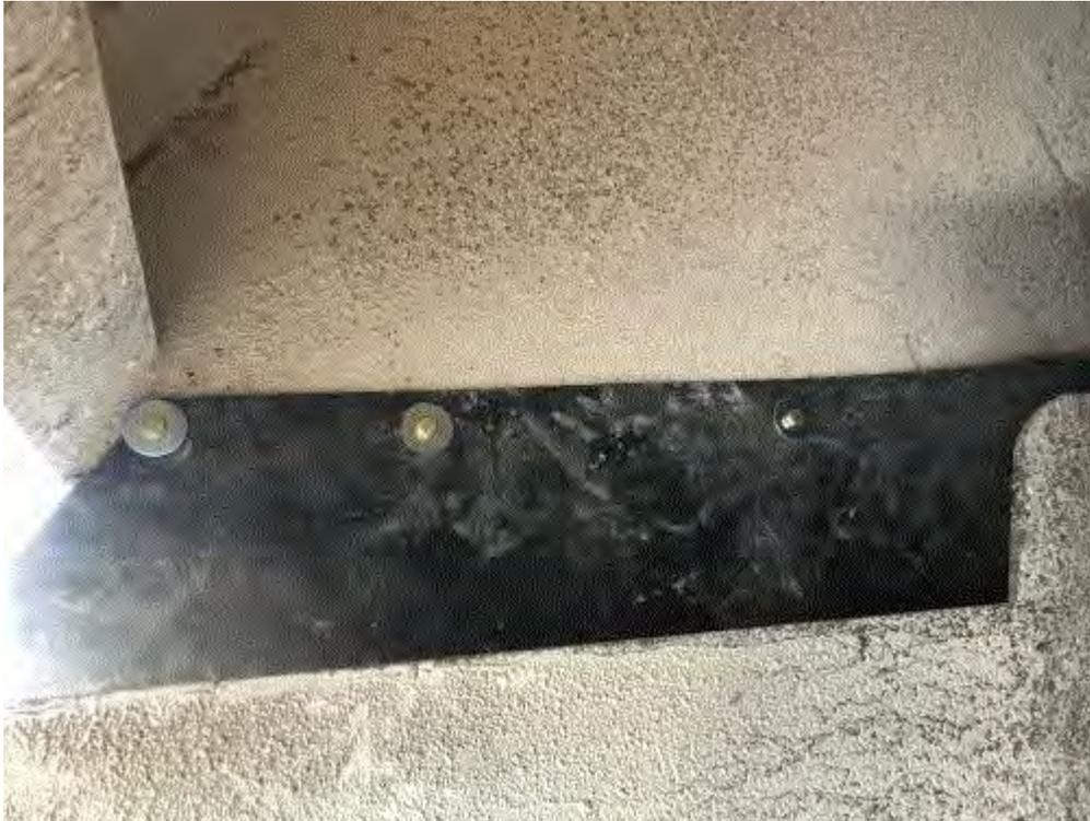
**Image 5(S1 Flashing)** : Flashing added to further enclose screen and minimize air intrusion
