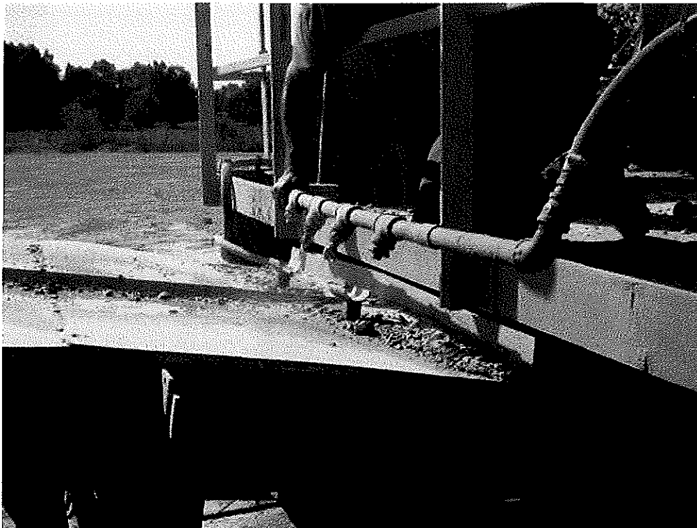
Image 5(Watersprays) : Conveyor watersprays
