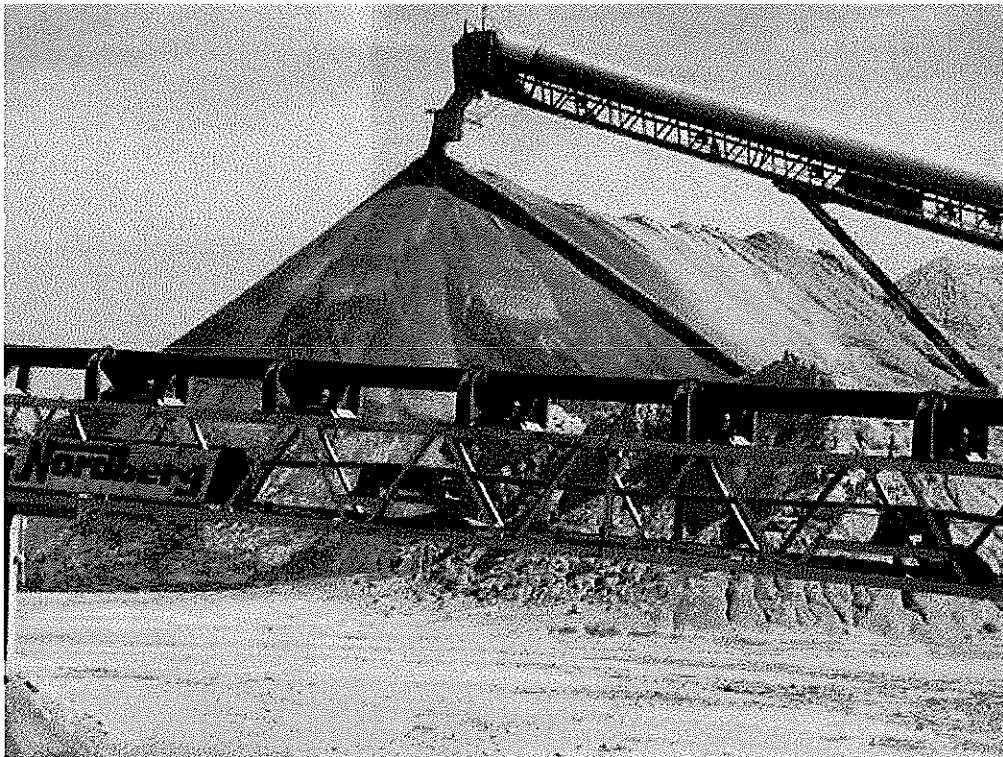
Image 9(Agg Lime Pile) : Equipped with boot at end of conveyor
