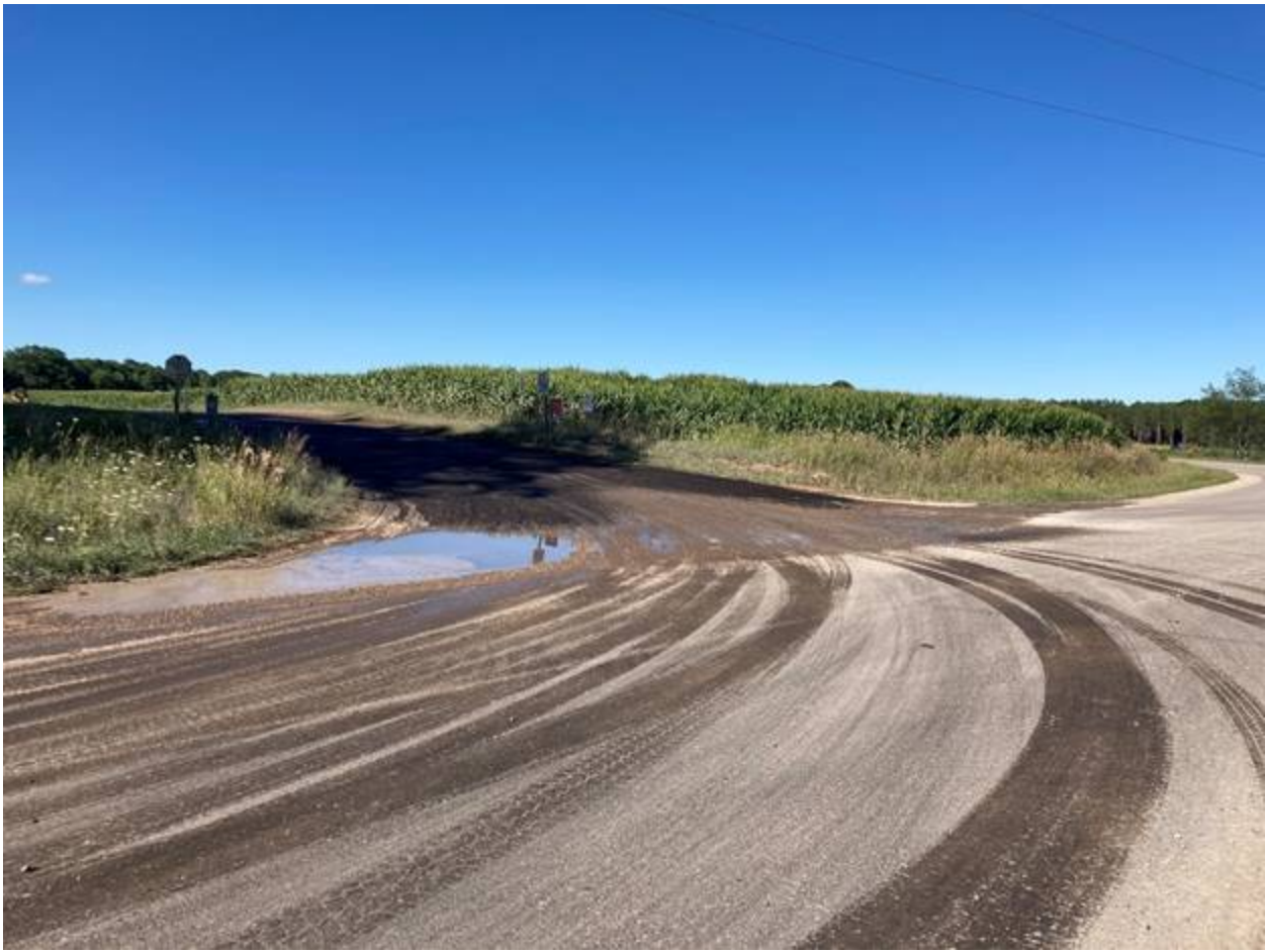
Image (6): Intersection after brine and asphalt applied.
