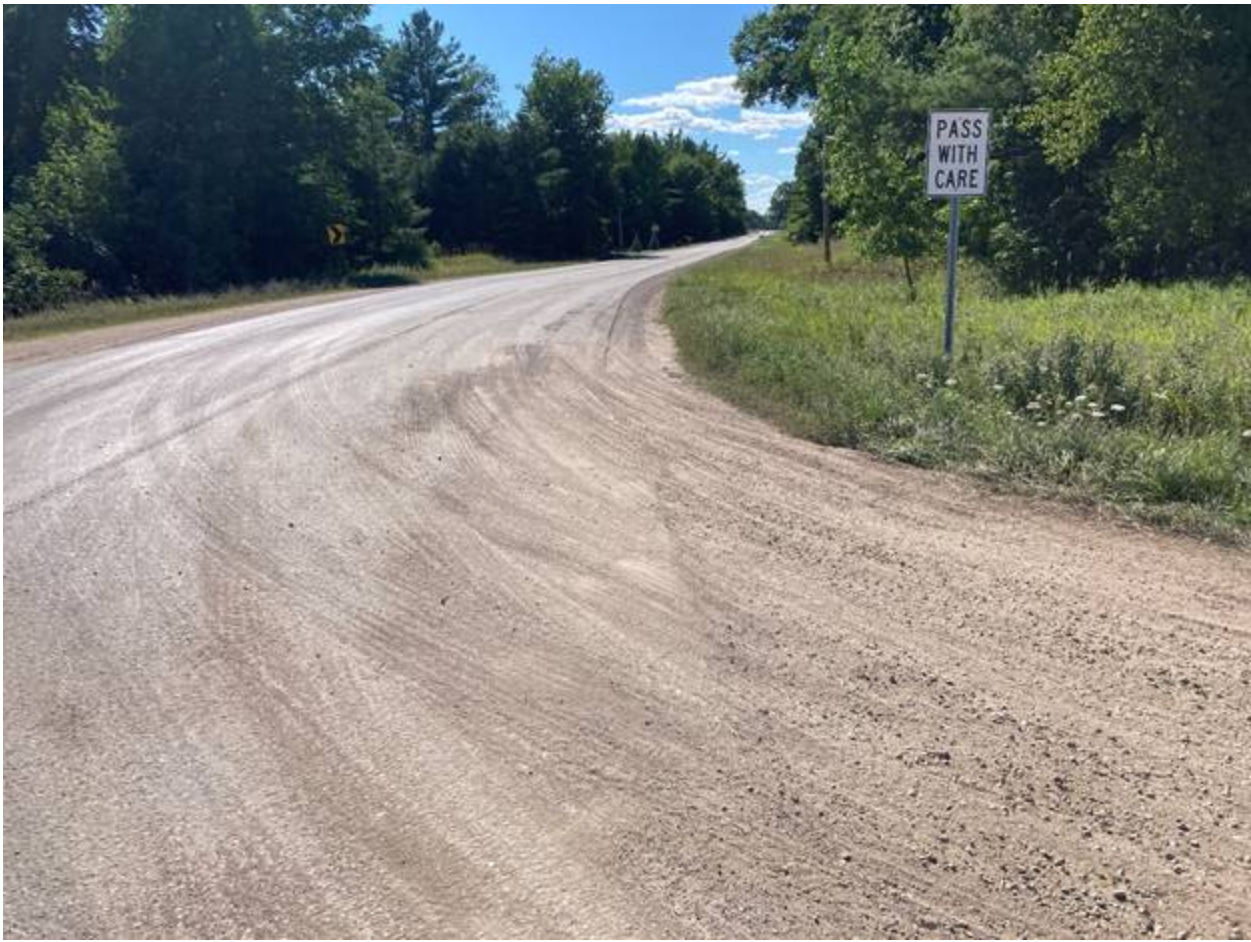
Image (4): Track-out observed onto County Road 338.
