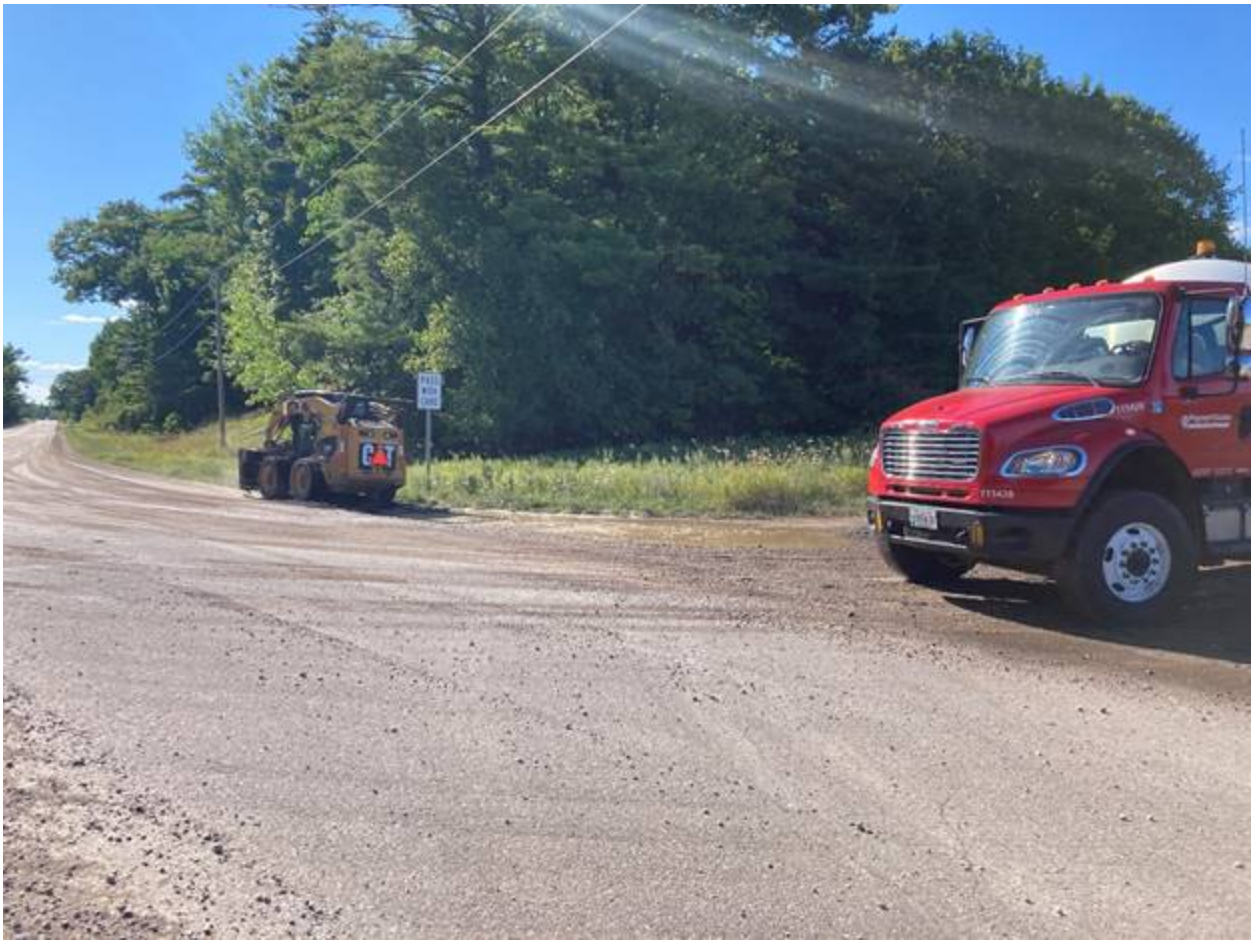
Image (5): Brine and asphalt being applied to the intersection.
