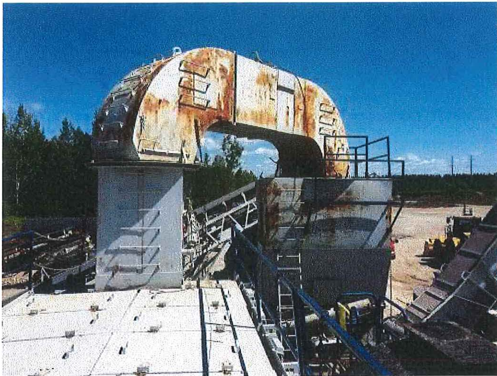
Image 3(Duct Work) : Duct work from dryer to baghouse.
