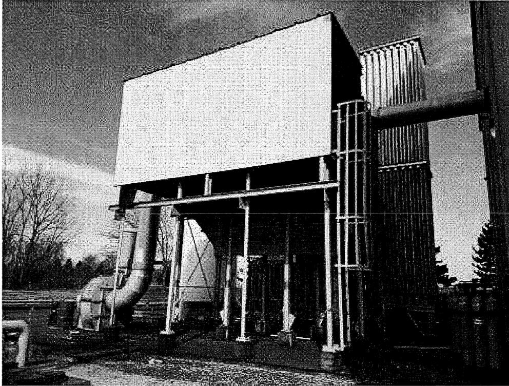
**Image 6(main dust collector)** : Main dust collector for furnaces. Stack exhaust can be seen on the ground to the left of the collector.
