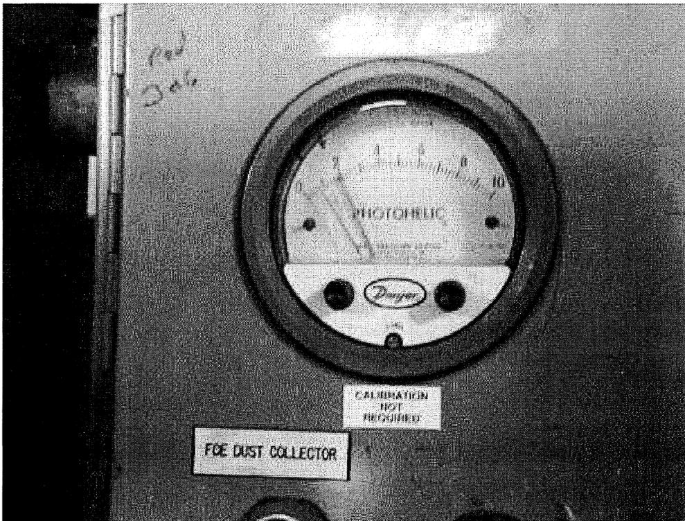
**Image 7 (pressure gauge)** : Pressure gauge for main dust collector
