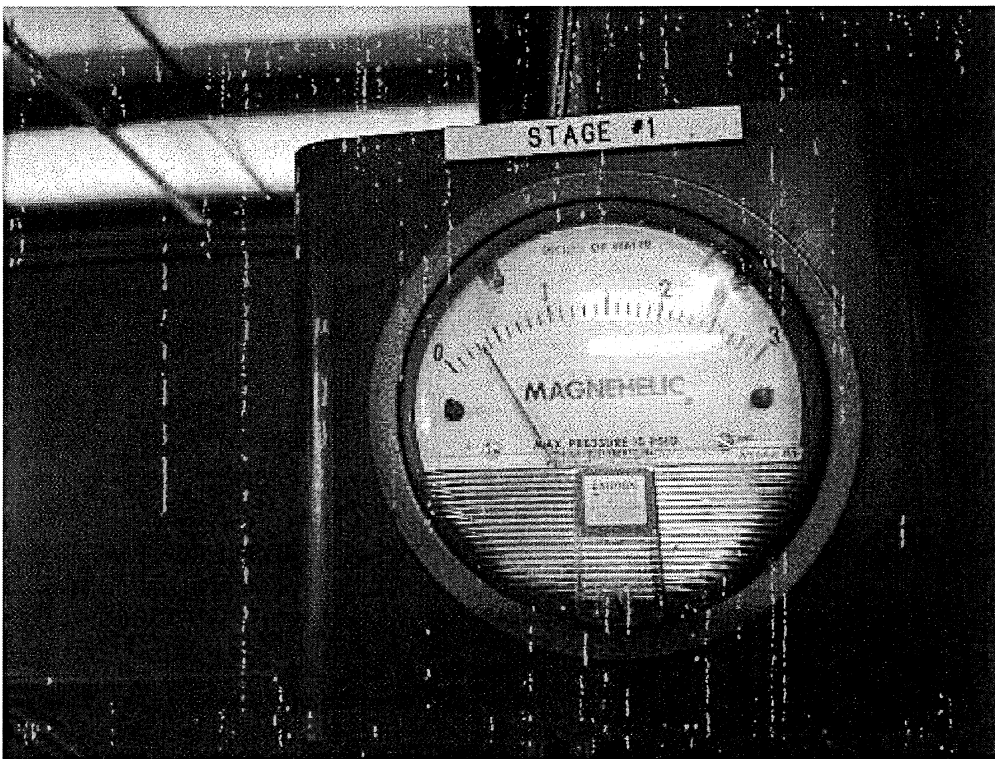
Image 8(B5 Stage 1 Scrubber) : B5 Stage 1 Pressure drop across the first mesh pad.
