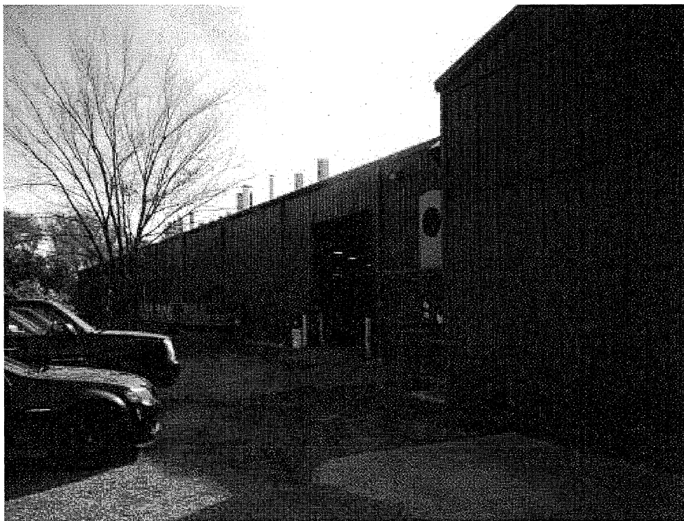
Image 1(Figure 1) : One of 2 bay doors located on the facility's western side. Emissions, generated from the heat treat lines, were escaping underneath the top of the door opening. 10/23/15, 11:25 am.
