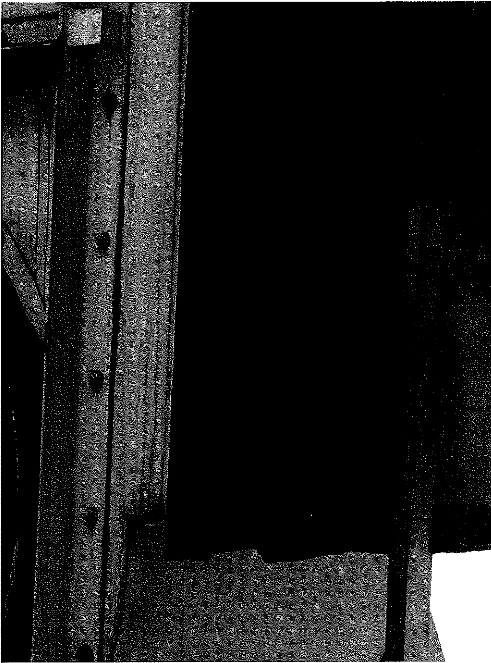
Image 2(Seal closup) : Missing seal.
