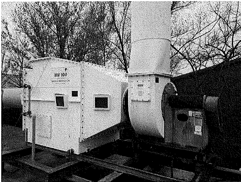
Image 2(Number 1 Scrubber) : Number 1 Scrubber. (Older)
