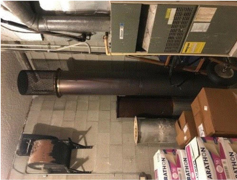
**Image 2(Stack) :** The dismantled stack where unit once was. Ceiling can be seen to have been closed since removal of stack.
