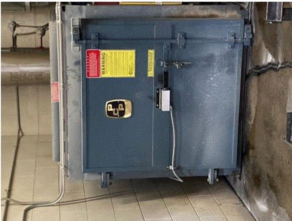
Image 2(Burn off oven) : Image of burn off oven installed in 2019
