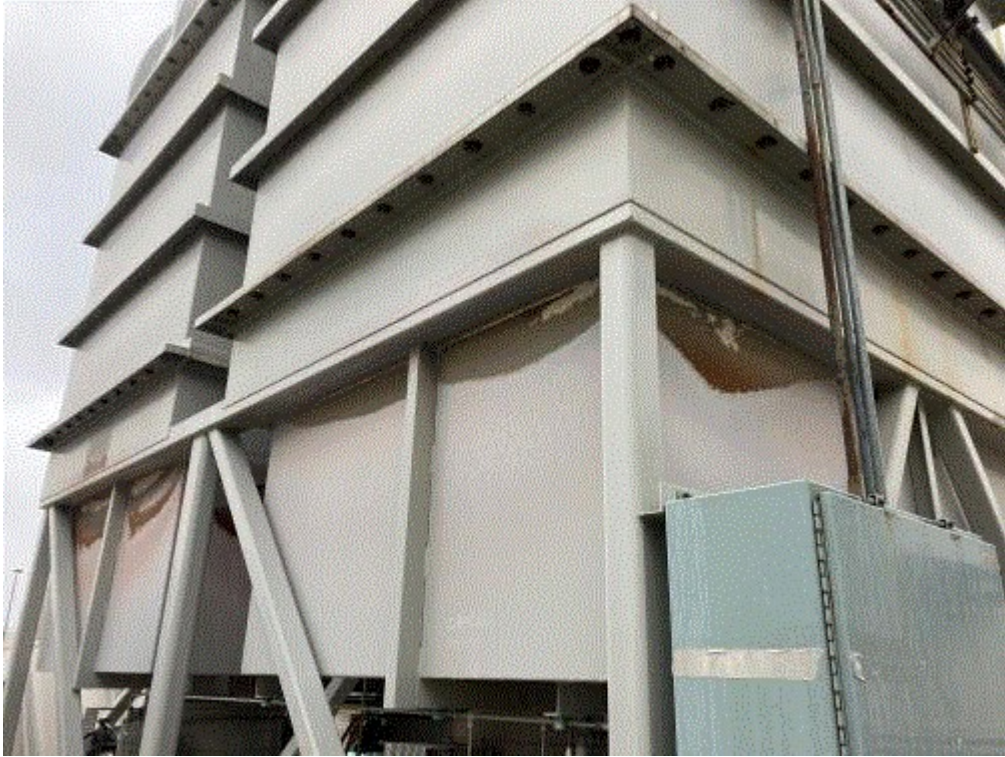
Image 1(Mirrors Oxidizer) : Photo shows paint wear on sides of unit.
