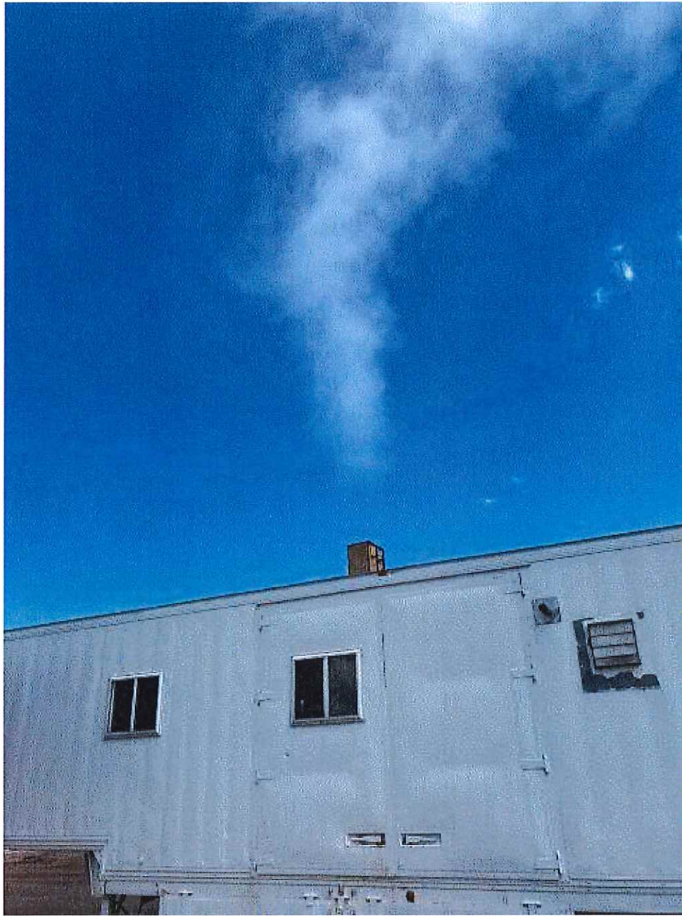
Image 1(Bacco Plant 12 Stack) : Steam coming from Bacco Plant 12 while operating
