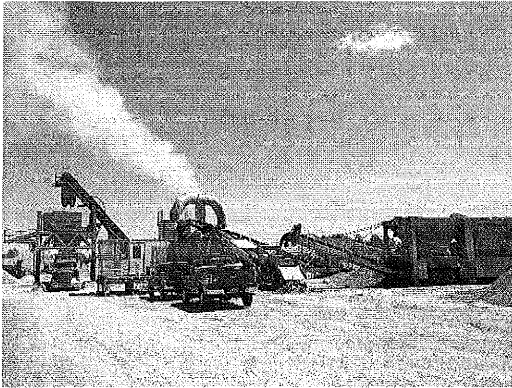
Image 3(7/24/2014) : Portable asphalt plant 25 spread.
