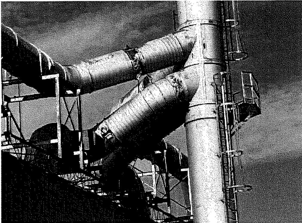
**Image 2(central stack)** : view of stack and wyse joints for central stack. Note the metallic coating of rubber banding at joints is coming off.
