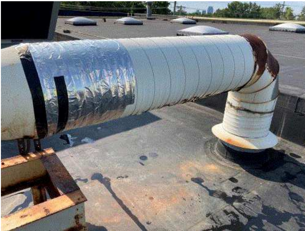
Image 1(FGWESTPOWDER Duct 1) : Image of FGWESTPOWDER Ductwork prior to fixing. Photo 1.
