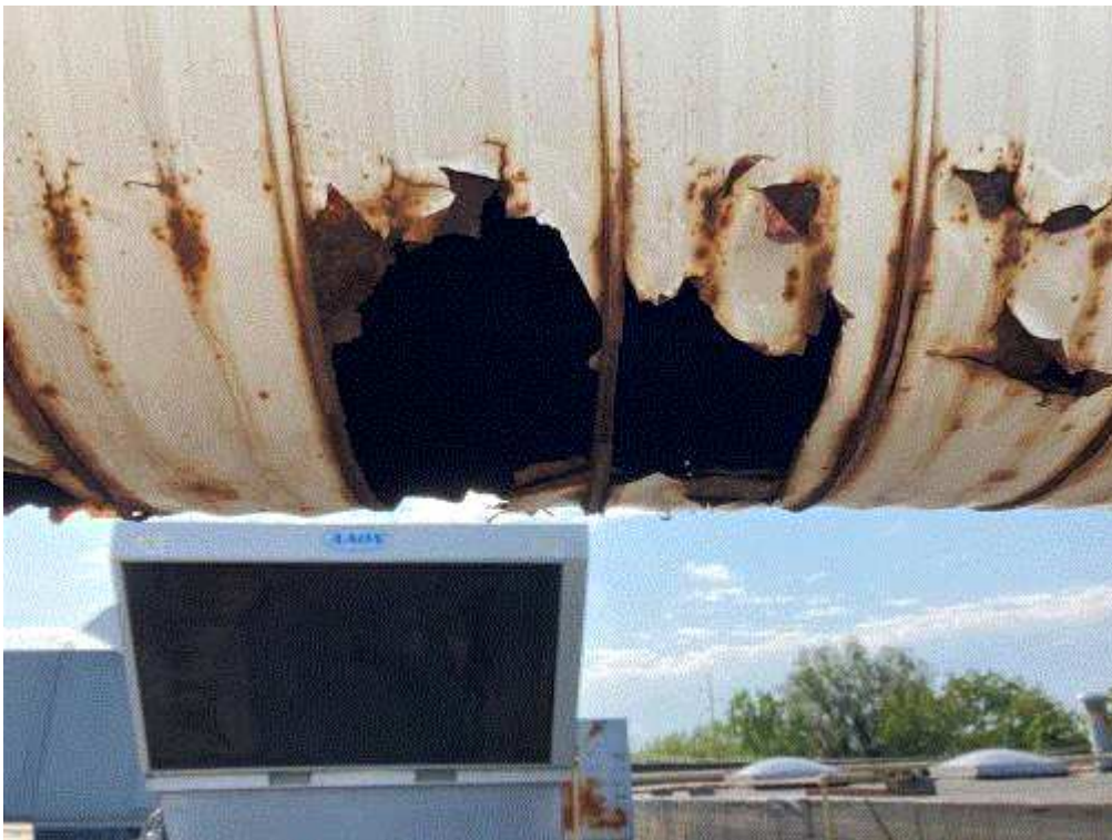
Image 2(FGWESTPOWDER Duct 2) : Image of FGWESTPOWDER Ductwork prior to fixing. Photo 2.
