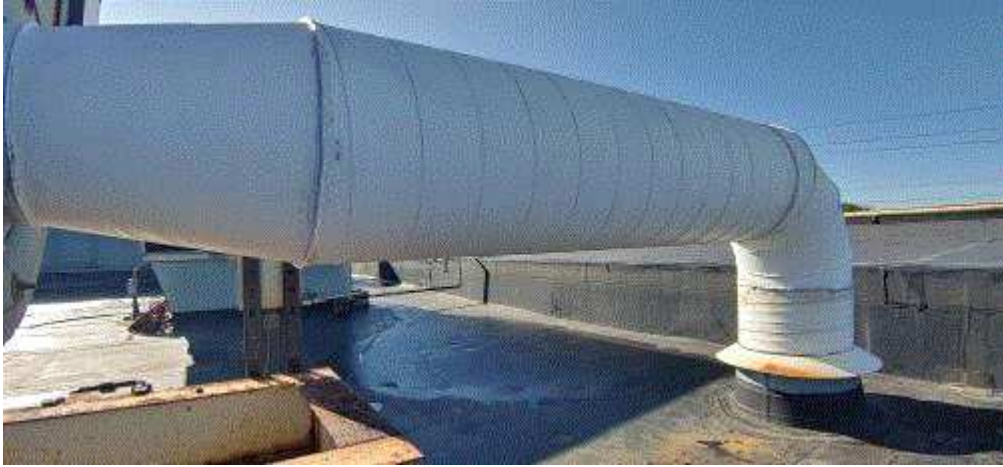
Image 3(FGWESTPOWDER Duct 3) : Image of FGWESTPOWDER Ductwork after replacement. Photo 3.
