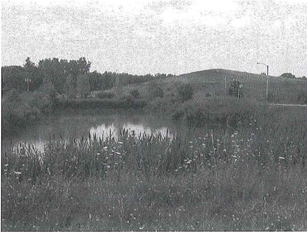
Image 5(storm water pond) : The storm water pond at the east end of the facility with the leachate pumping apparatus and the ash monofill in the background.
