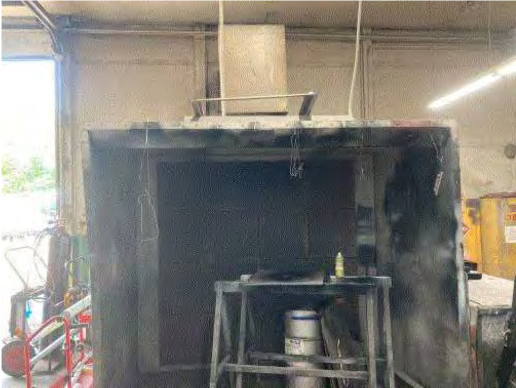
Image 4(IMG_0248) : Small paint booth
