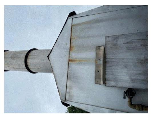
**Image 1(REPAIRED FACIA):** Image from permittee demonstrating repair of triangular exterior panel.
