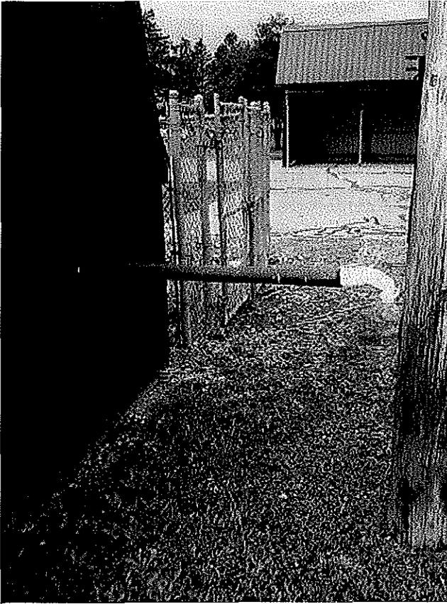
Image 1(Stack Pipe) : Pipe was once attached to a stack. Stack has been removed.
