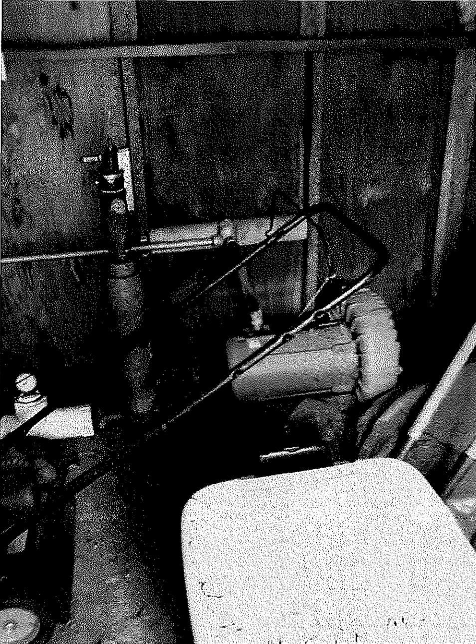
**Image 4(SVE System) :** Component of the SVE system which is attached to the pipe protruding out of the north side of the shed, once leading to the stack.
